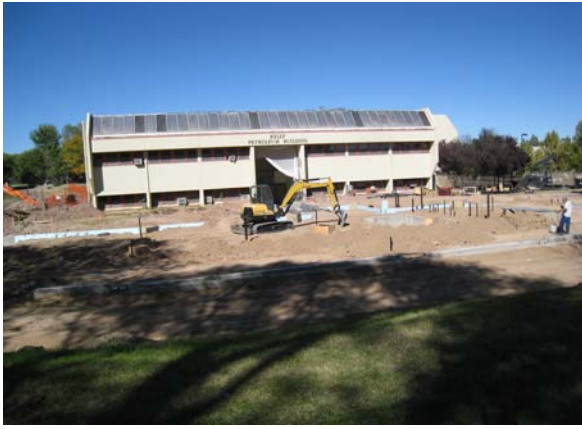
PRRC Construction, October 2008
